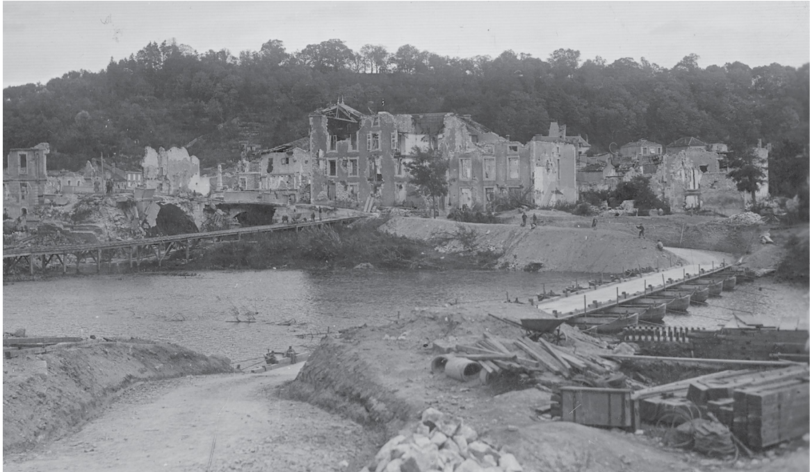
St. Mihiel Soon After Its Capture; Note ponton bridge built by American Engineers
