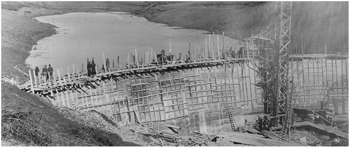
Storage Dam at Savenay Being Constructed by American Engineers
