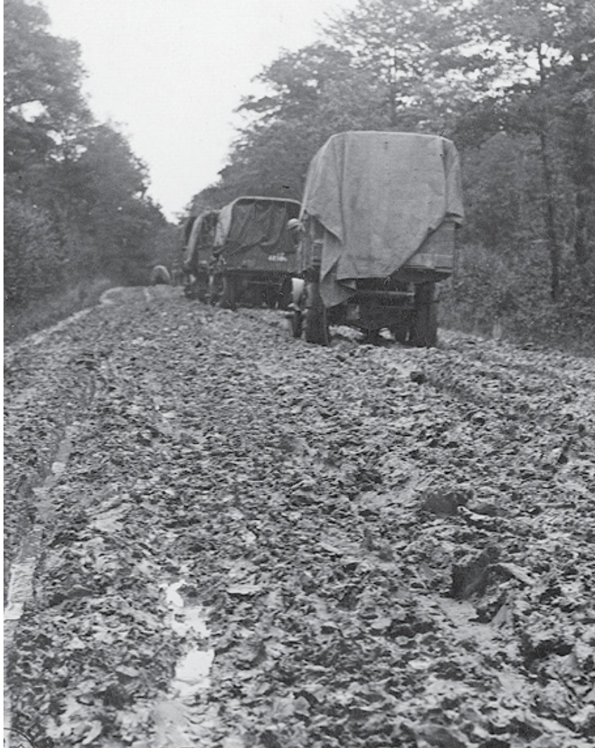
Road Near Sanzey Just Before the St. Mihiel Offensive: Note its muddy, torn-up condition typical of most roads in the region at that time
