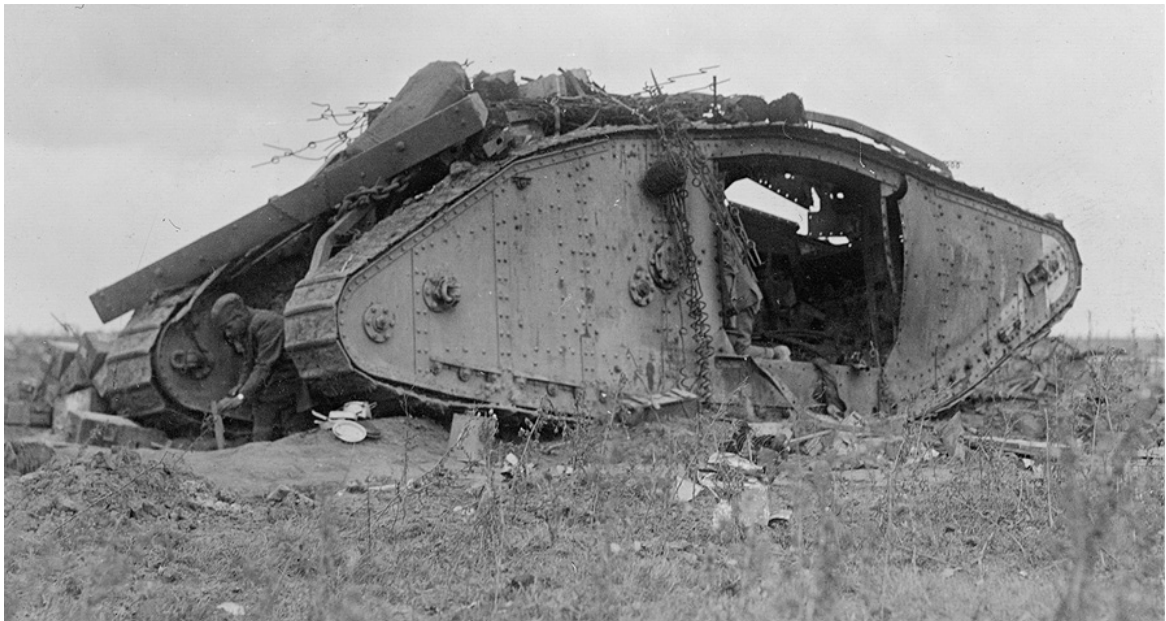
27th Division Tank Destroyed by a German Mine East of Ronssoy
