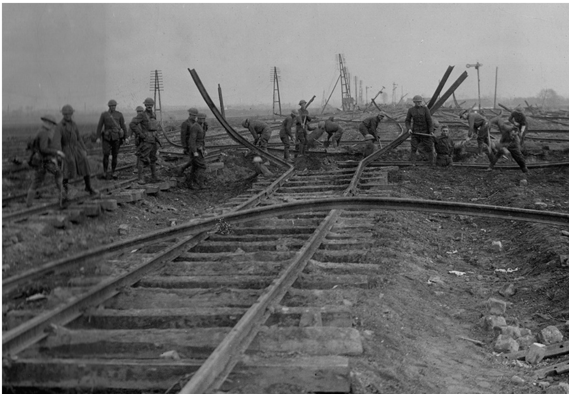
91st Division Engineers Repairing Tracks Blown Up by the Germans Near
