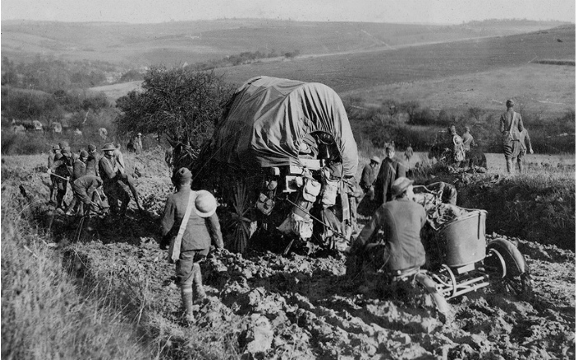
Engineers Working on Road Near Barricourt, November 4, 1918, Note condition of road
