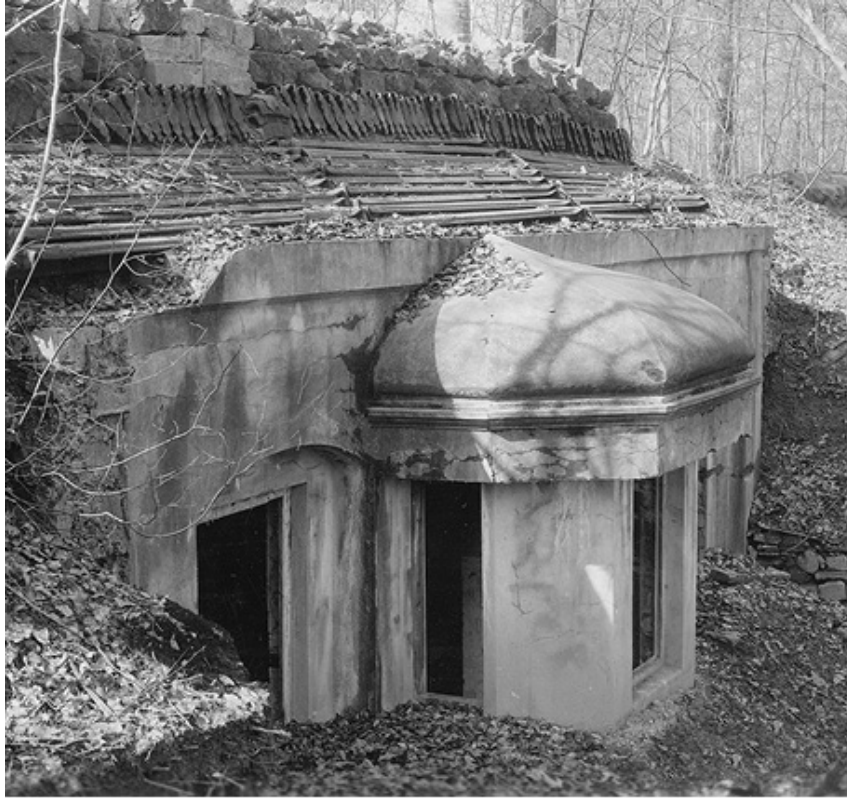
Concrete Dugout in Champ Mahaut
