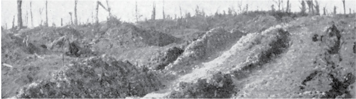
Results of Traffic on the Avocourt–Malancourt Road Built Over No Man's Land
