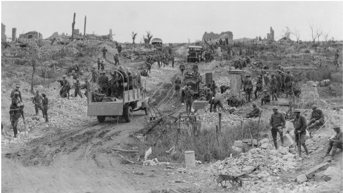
90th Division Engineers Repairing Road at Fey-en-Haye, September 1918
