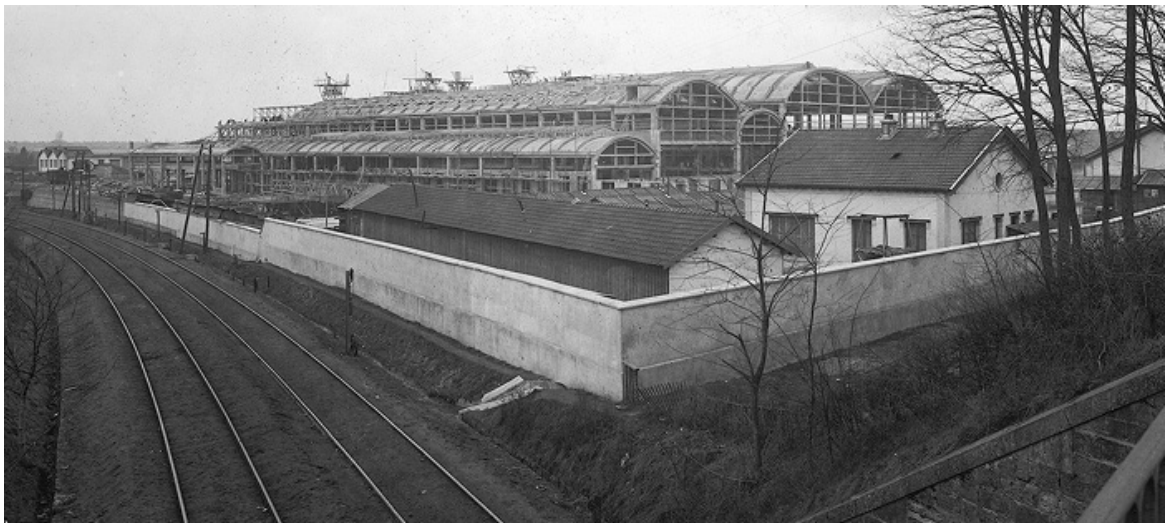
Locomotive Repair Shop at Nevers Under Construction by American Engineers. Nevers was an important railroad and storage center
