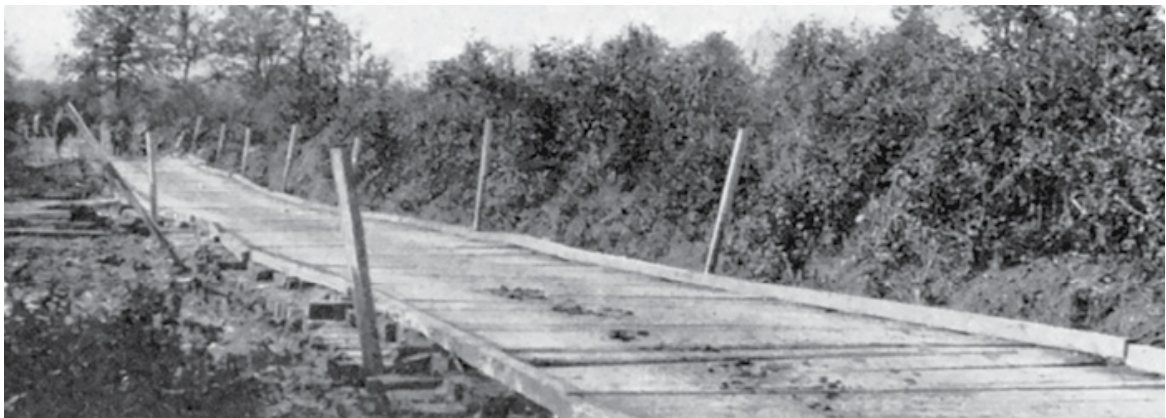
Section of Avocourt–Montfaucon Road Showing Plank Construction
