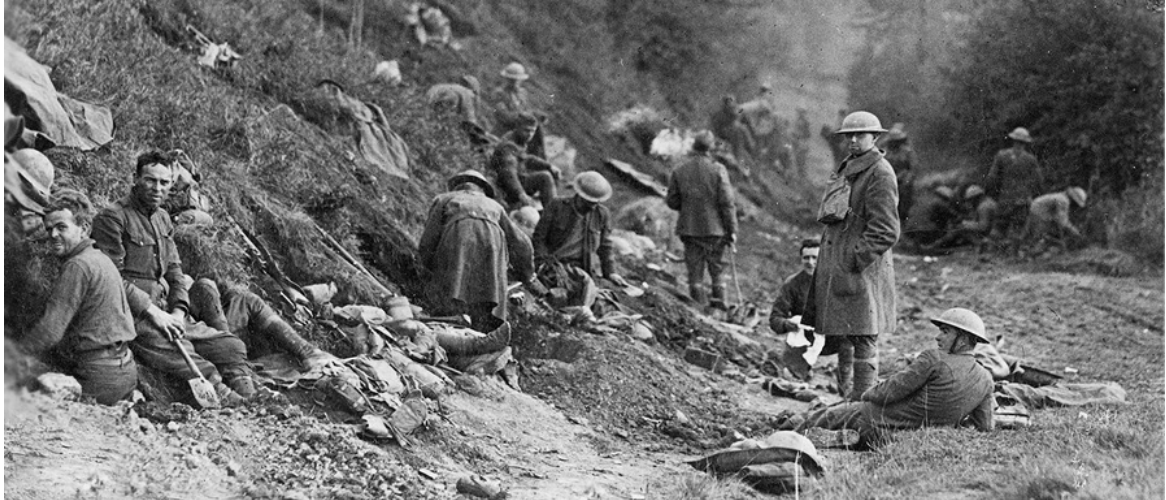
30th Division Reserves Digging In Near Molian, October 18, 1918
