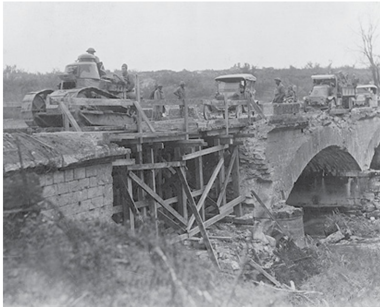
Bridge at Boureuilles After Repairs Had Been Made, September 28, 1918
