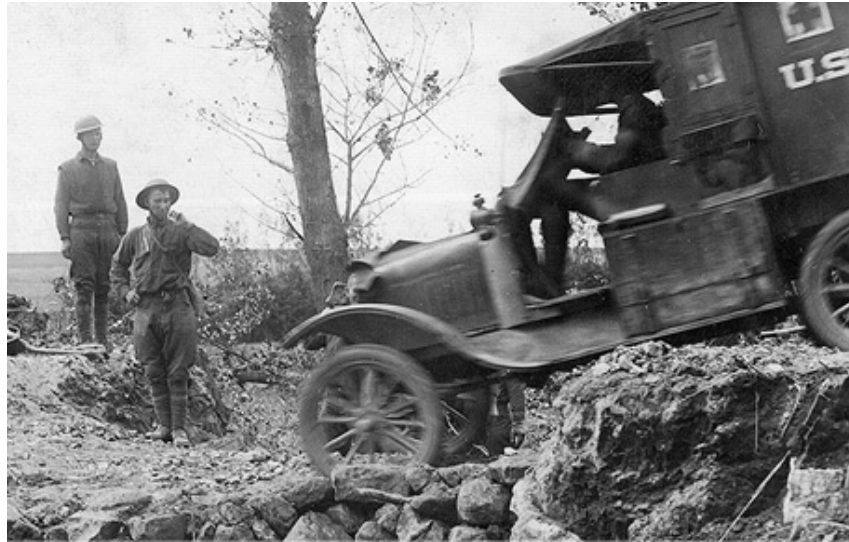
The Repairing of Roads Was a Problem for the Engineers
