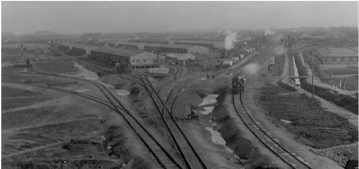
Railway Yards and Warehouses at St. Sulpice Constructed by American Engineers
