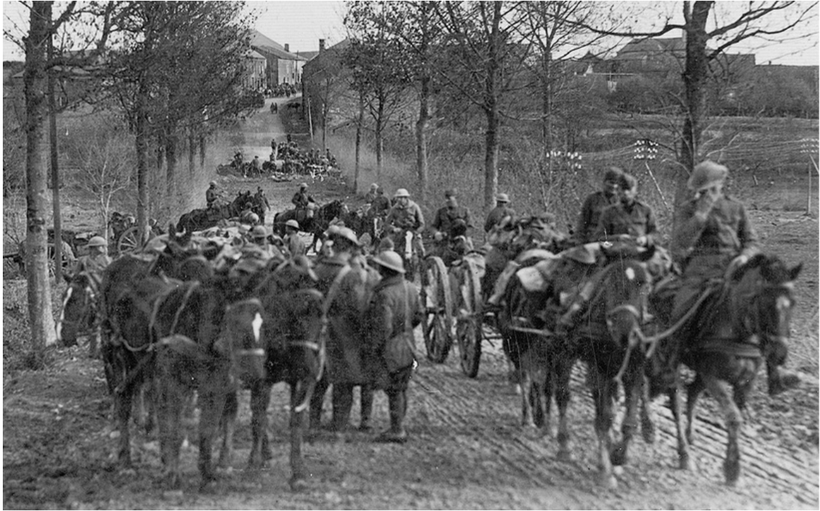
Troops West of Bar, Compelled to Pass Around Bridge Being Repaired, November 3, 1918
