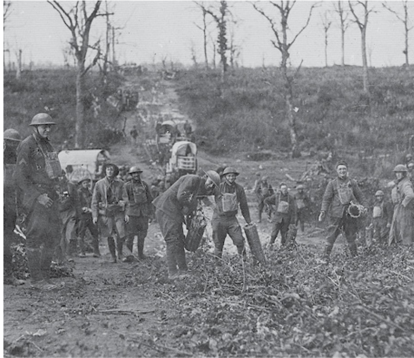
37th Division Engineers Repairing Road Near Montfaucon, September 28, 1918
