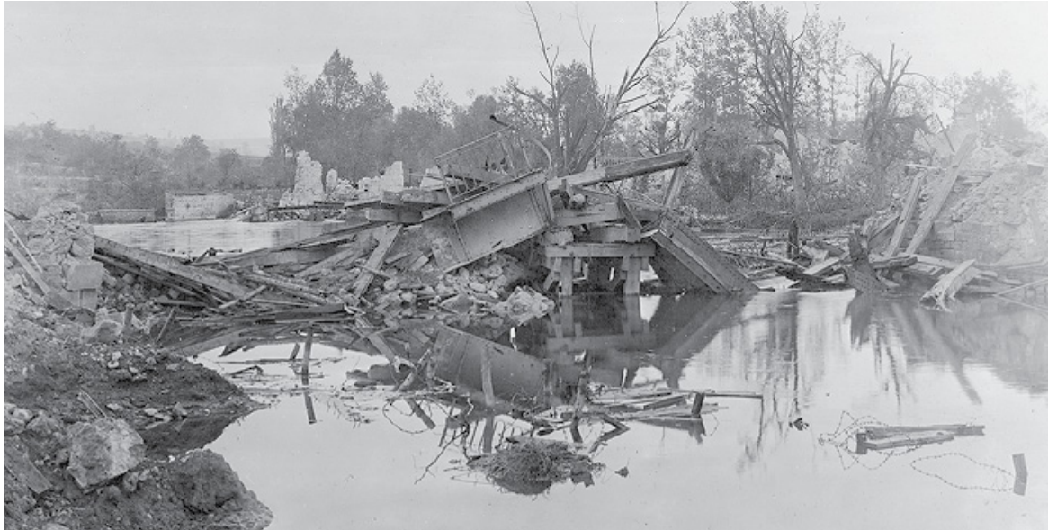
Main Bridge Between Fismes and Fismette Destroyed by the Retreating Germans
