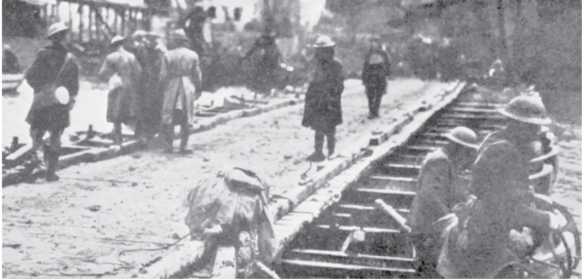
Ponton Bridge Constructed by 5th Division Engineers Near Dun-sur-Meuse
