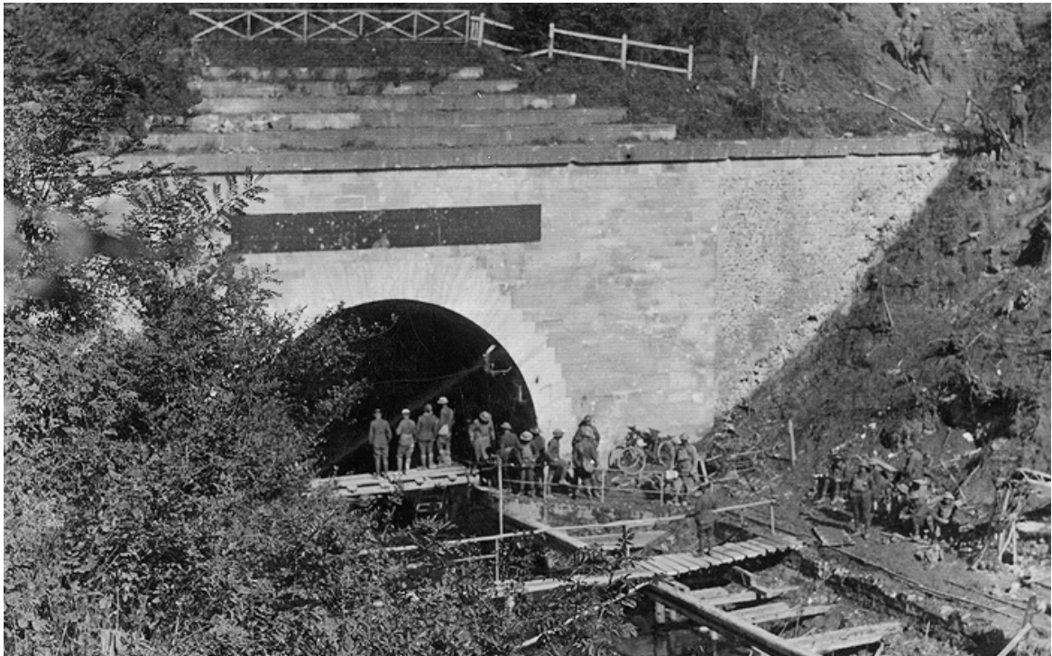
Southern Entrance to the St. Quentin Canal Tunnel, Near Bellicourt, October 1, 1918
