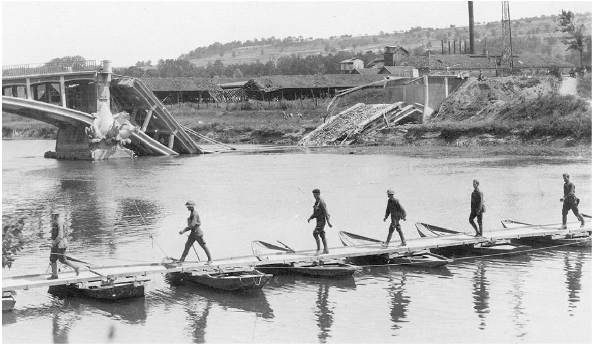
Ponton Bridge Near Mézy Built by Engineers of the 3d Division
