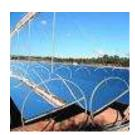
Aus ra is at the vanguard of large scale power generation. Its solar storage system generates power at centralized stations using concentrating solar power to create steam that turns a turbine to make electricity. It also stores hot water that a power plant can draw on during times when the sun is not shining, reducing the cost to 8 cents per kilowatt hour, compared to 12 cents for natural gas. http://www.ausra.com/
