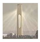
Solucar 600-mirror Solar Tower in Seville Spain is the first commercial concentrator station in Europe. It focuses Sunlight onto water pipes at the top of a 40-storey concrete tower, which drives a turbine to generate 11 megawatts of electricity. Thousands more mirrors will be added to further boost the output. Added details: http://www.solucar.es/
